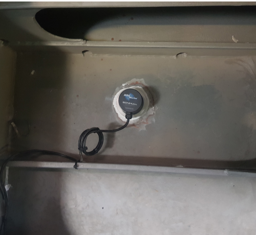
Photo 3: An ultrasonics transducer fixed to a ships' hull
