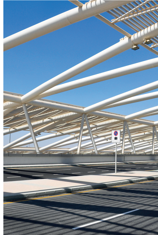
Cairo International Airport, Terminal 3 – protected by SteelMaster
